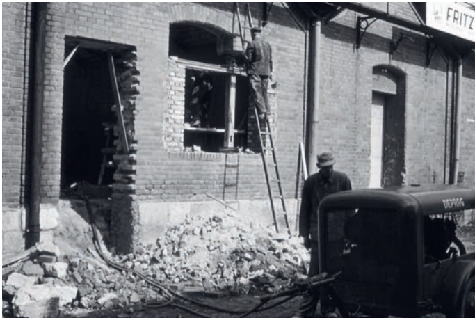
Construction of the business premises in the Gasfabrikstraße
